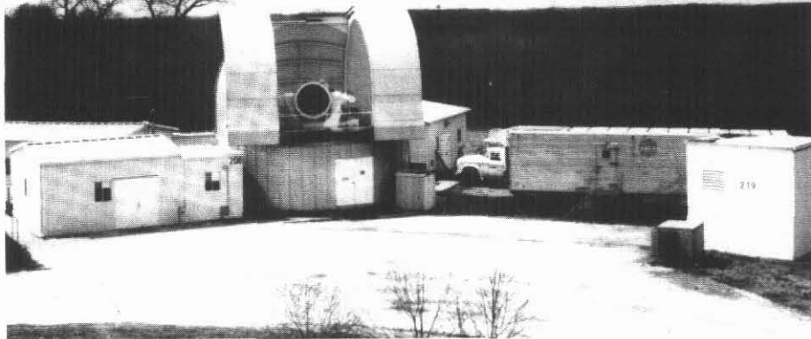
Figure 5. 1.2-meter telescope. The laser is in the structure beneath the telescope. The building at left contains the telescope tracking computer. The building in rear contains the stationary maser and event timer and electronic equipment. The water tower is visible on the horizon.
